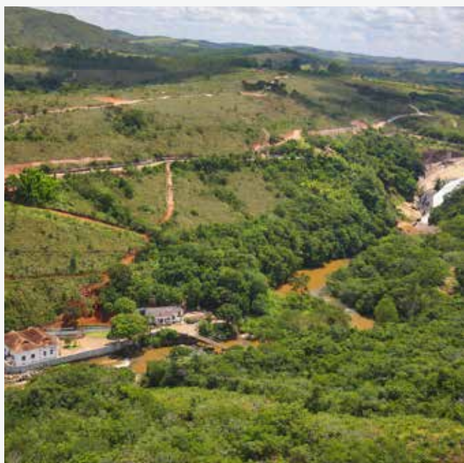
AMG hydroelectric plant in Brazil
