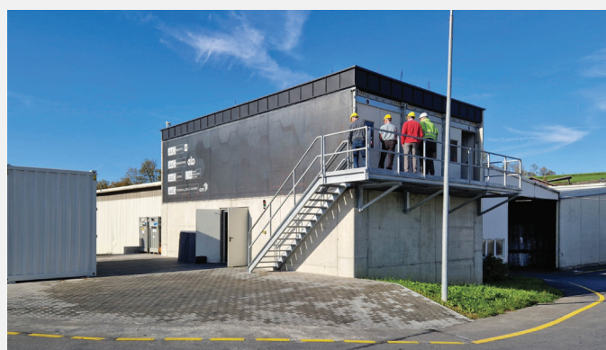
LIVA Power Management Systems GmbH - Frankfurt, Germany
