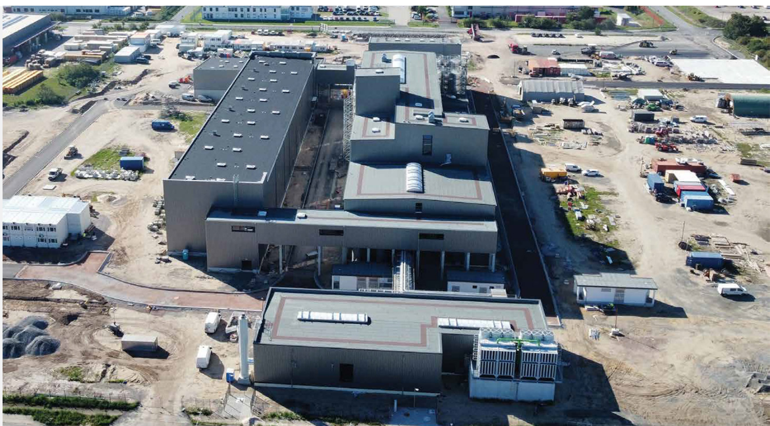
Lithium Hydroxide battery-grade refinery - Bitterfeld, Germany
