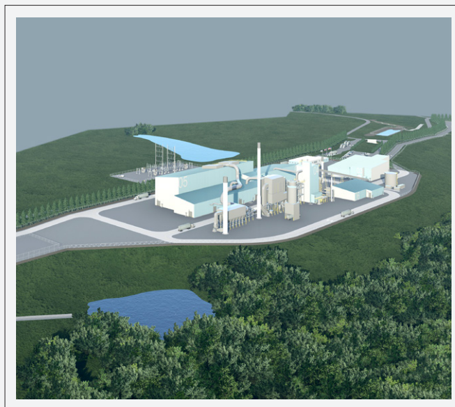
ZANESVILLE, OHIO PLANT (UNDER CONSTRUCTION)
