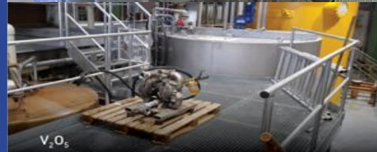
MELTSHOP - ZANESVILLE, OHIO
