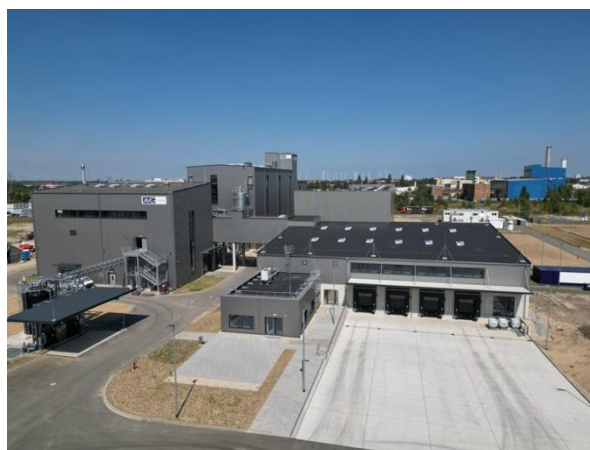
AMG Lithium, Lithium Refinery, Bitterfeld-Wolfen, Germany
