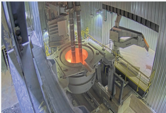
AMG Vanadium - Zanesville, Ohio, USA facility meltshop
