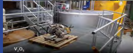
MELTSHOP – ZANESVILLE, OHIO
