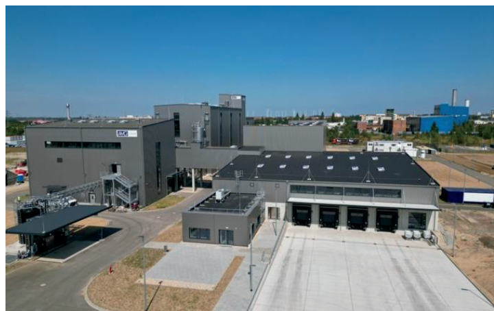
📍 AMG Lithium, Lithium Refinery, Bitterfeld-Wolfen, Germany
